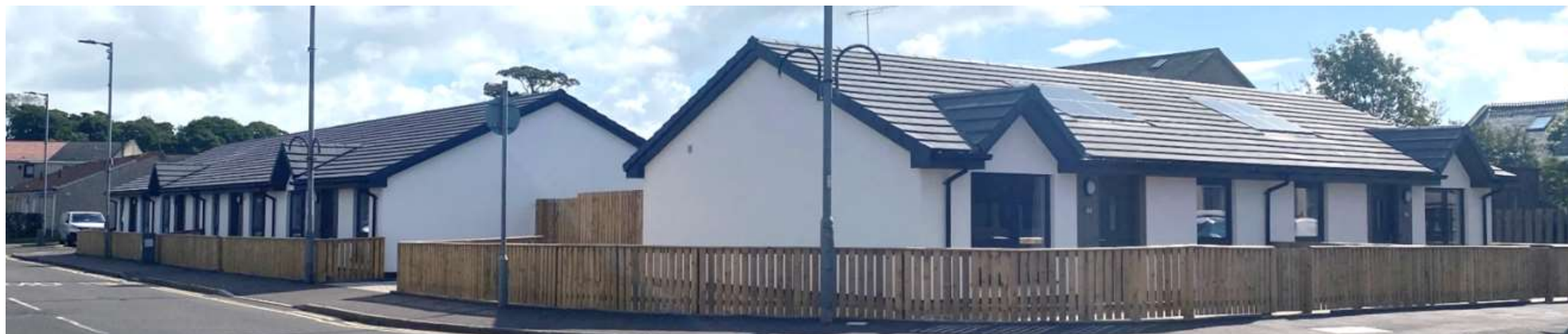
Figure 4: Afton Court development of six amenity bungalows utilising off site construction in Stevenston town centre
