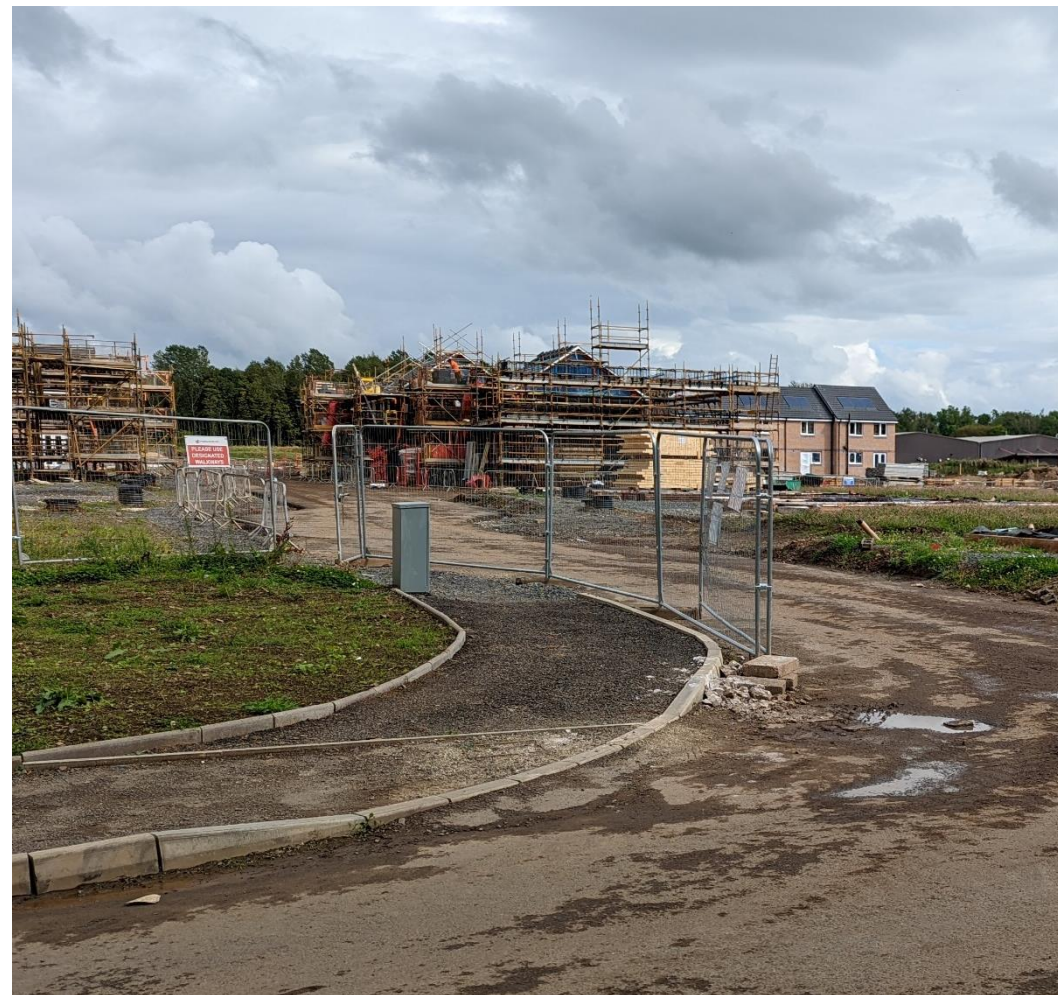
Housing on a previously derelict site at North Newmoor, Irvine
