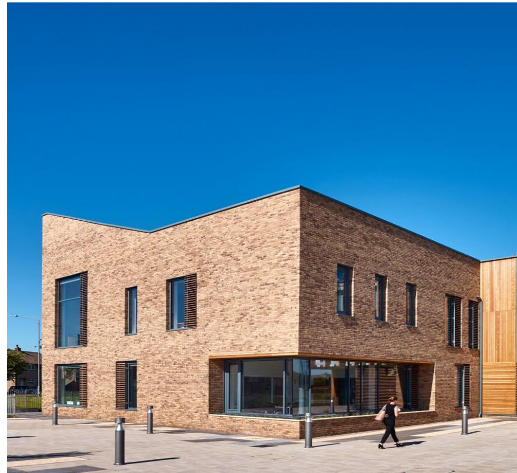
Quarry Road, Irvine.
