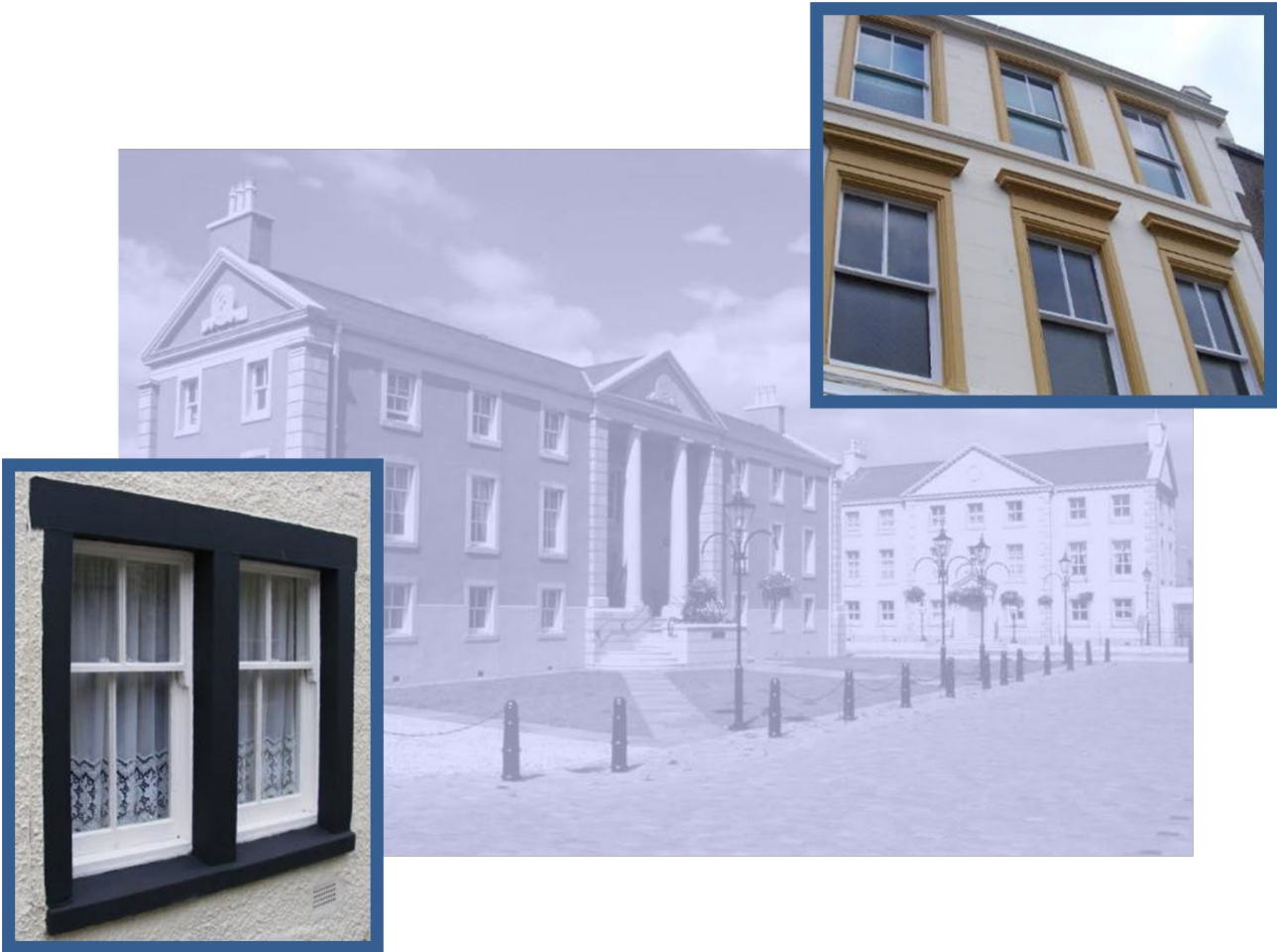
Figure 2 - Examples of timber sash and case windows
